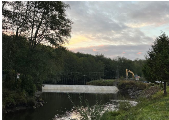
The Makah NFH fish weir after repairs.
