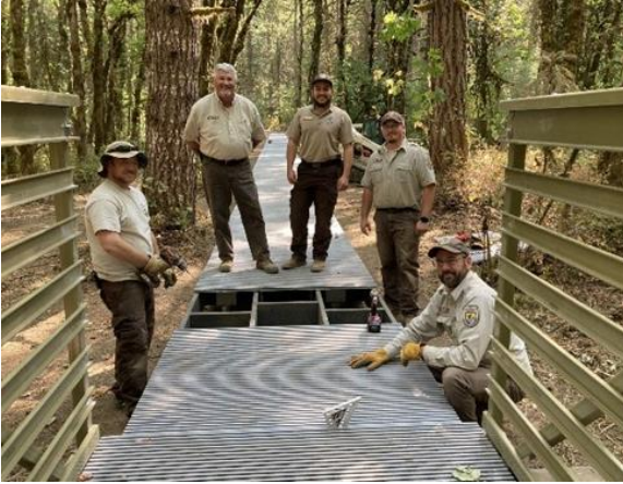
GAOA MAT Strikeforce Team Members Constructing a Replacement Accessible Trail Bridge at the William I. Finley NWR. Credit: USFWS
