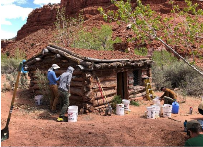
Volunteers work on restoring the roofing and chinking of Watson Cabin.
